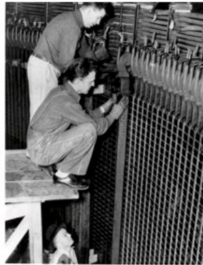
Stator and Rotor of Synchronous generator of Grand Coulee hydroelectric power plant on the Columbia River in Washington State.
