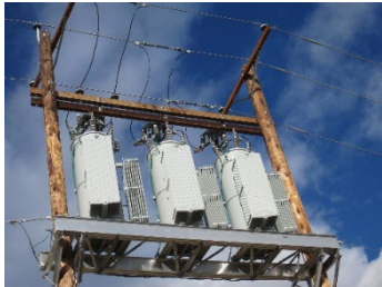
Load tap changer Voltage regulator Capacitor bank
